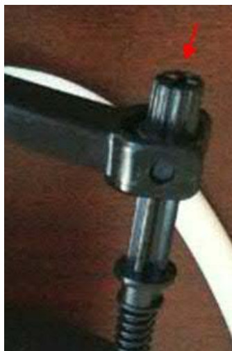
How to adjust floating cup (water level inside the tank) (Figure 2)
