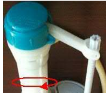
Turn valve body 1/8 turn counter-clockwise (Figure 5)
