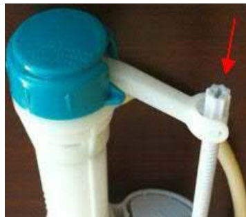
How to raise water level or lower it inside the tank (Figure 3)
