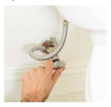
Step 2 - remove supply line from fill valve shank
