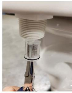
Step 4 – Check filter for debris. If debris is found clean out filter and wipe out the inside of the shaft to remove debris.
